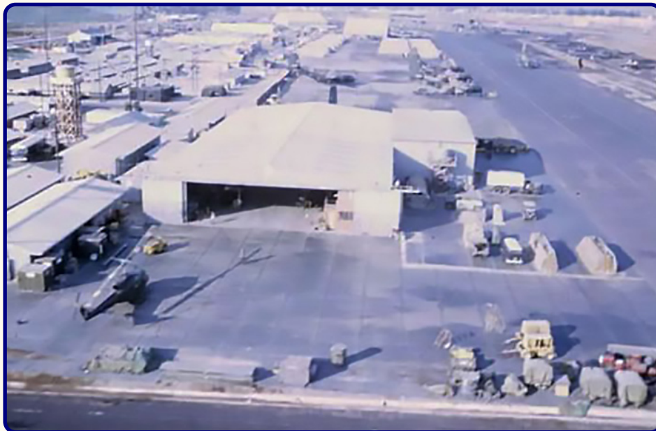
No. 9 & No. 35 Squadron hangar at Vung Tau airfield
