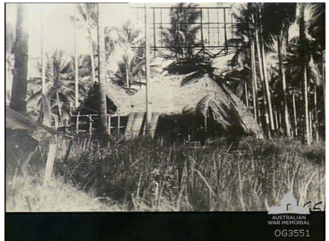
The 37 RS UK Mk V COL Radar with a simulated Papuan Hut constructed around it
